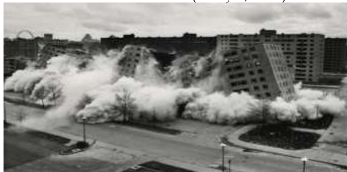
Figure 8: Minoru Yamasaki, Demolition in Pruitt-Igoe, Photograph, 1972, Missouri, USA . Source: Keskyes
