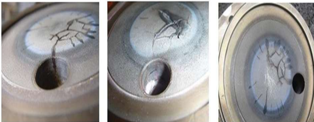
Figure 2: Gas turbine pilot burner crack.
