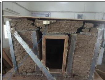
Fig 15 Collapse of Model A1
