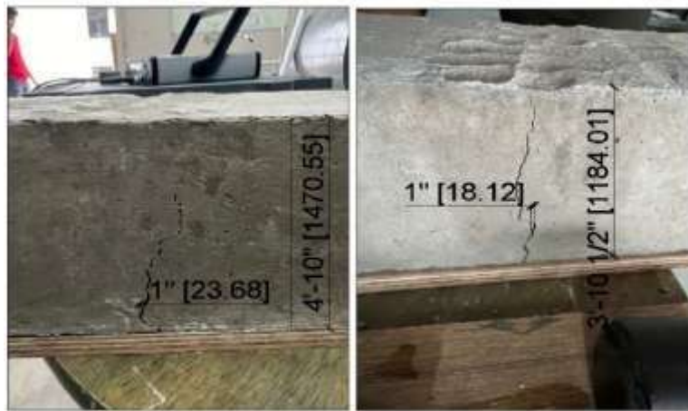
Figure 4. Post-crack loading of self-healing concrete (1.5% bacteria dosage mix) at 3 and 7 days.
