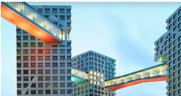
Figure 6. Skybridges Connecting 18 Level
