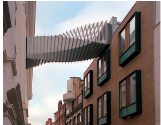
Figure 8. Bridge of Aspirations, UK
