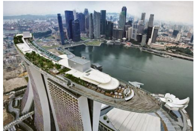
Figure 7. Marina Bay Sands Skybridge
