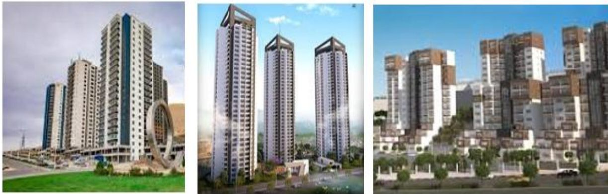
Figure.3: Barzayakany sulaimani project, Parck 77, Dayk Project- Sulaymanayah Housing projects /high-rise
