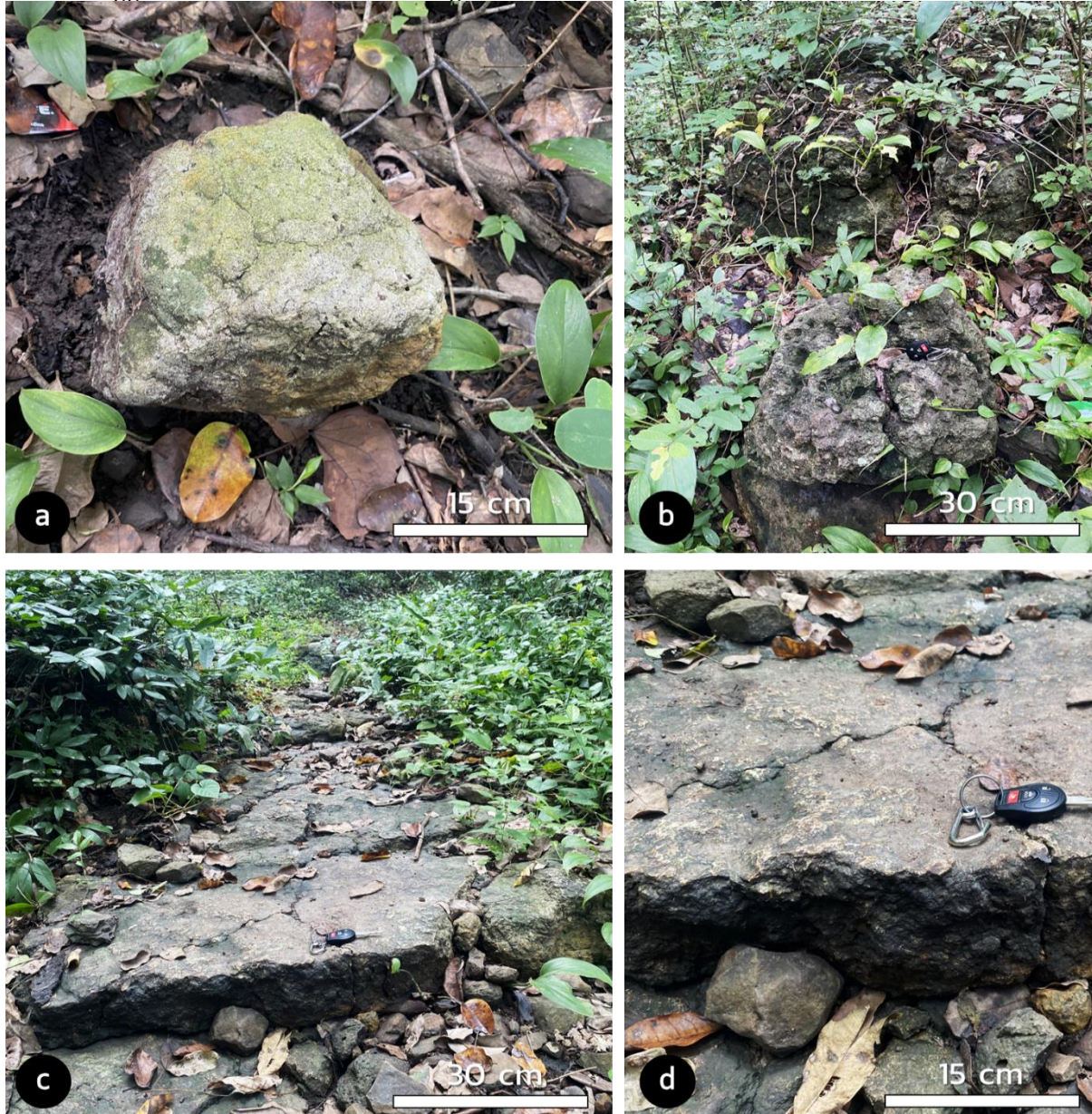
Figure 3: (A) Representative Sample of Anomalous Material Identified During Field Survey, Preliminarily Interpreted as Non-Basaltic in Origin and Visually Resembling Heavily Weathered Cementitious Material Resulting from Prolonged Exposure and Degradation. (B) General Condition of the Forested Surface Environment on PNR During the Rainy Season, Showing Anomalous Pale Material Recurrently Intermixed with Naturally Occurring Basalt Blocks Across the Forest Floor. (C-D) Flattened and Stepped Anomalous Surface Features Displaying Planar Morphologies Inconsistent with Natural Volcanic Landforms,
