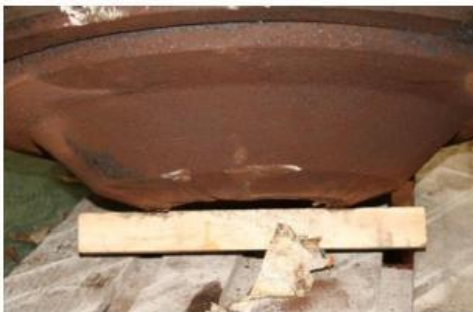
Figure 7: Corrosion of the inner face of the cover
