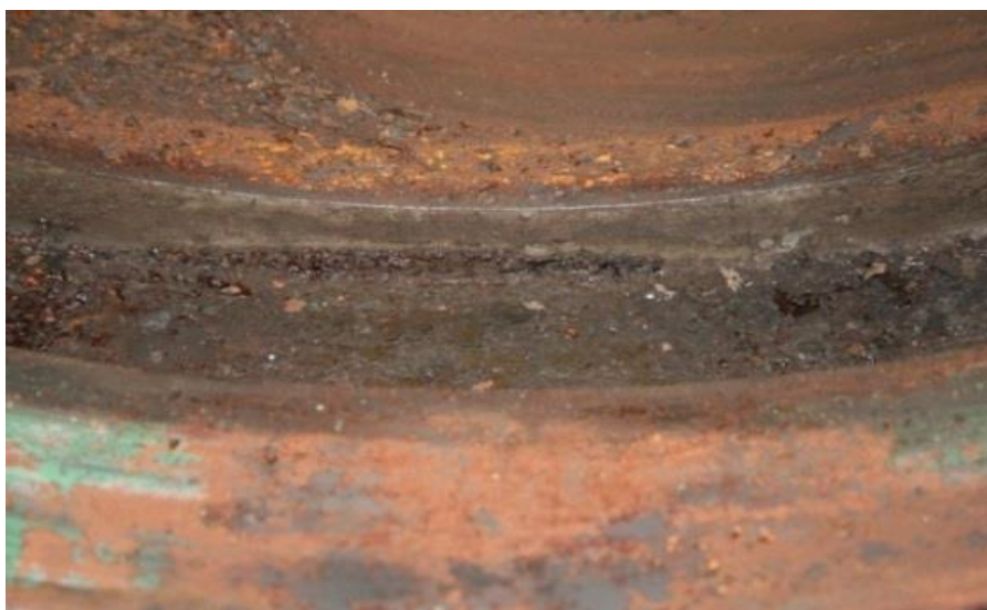
Figure 5: Corrosion of the shear ring groove
