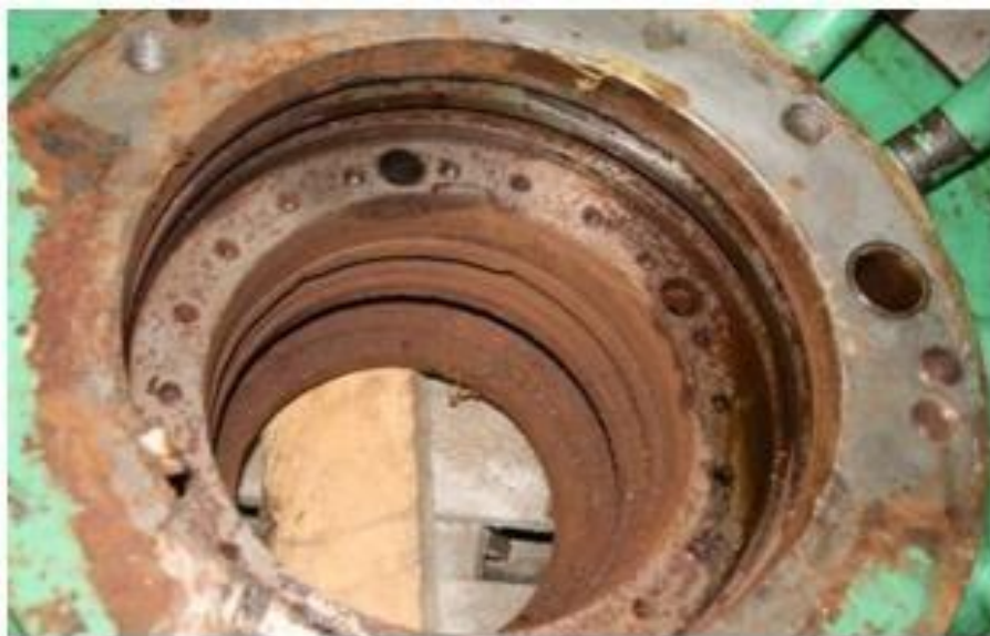
Figure 6: Corrosion of the cover seal location
