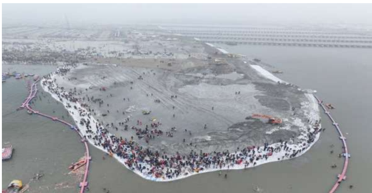
Figure 25: Historical Sangam Nose Reclaimed and Expanded by Dredging Process
