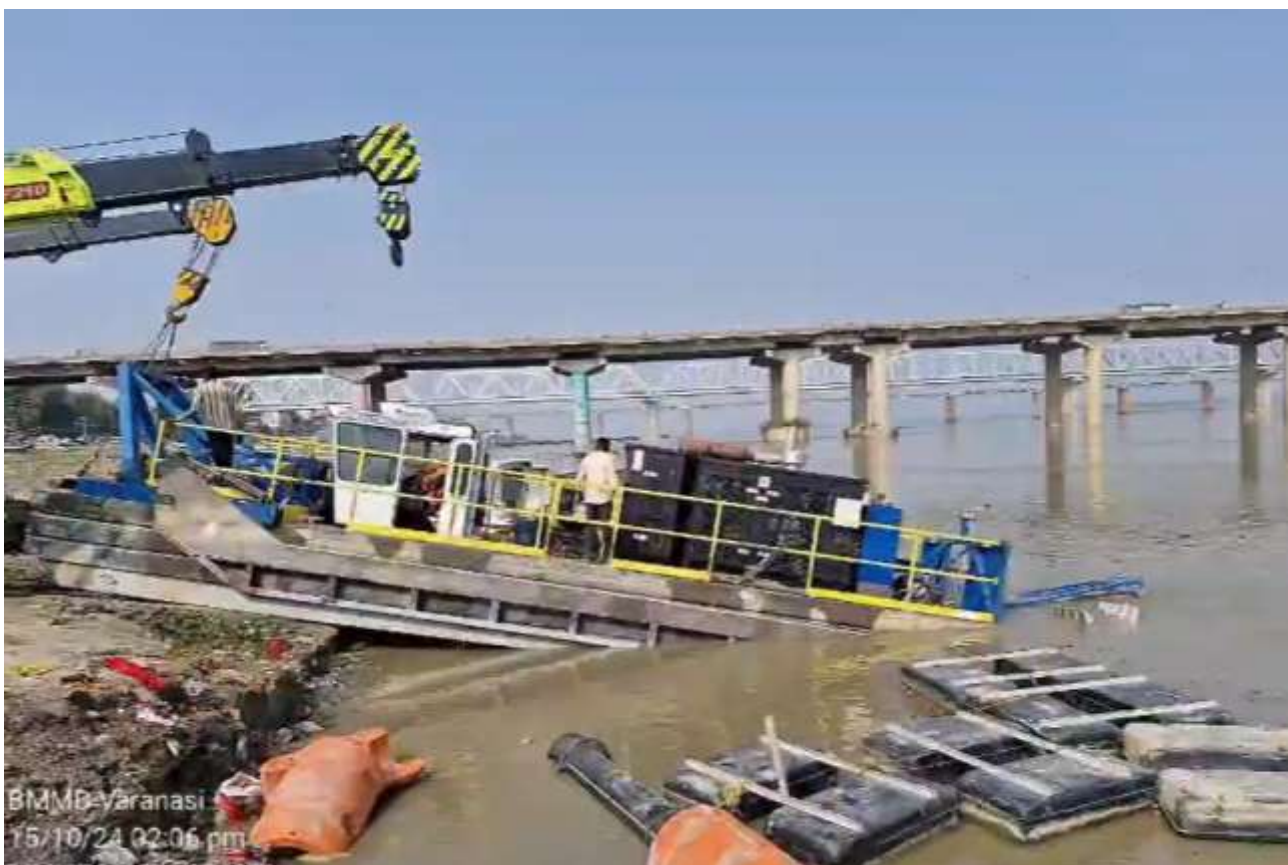
Figure 15: Launching of Dredger Machine in Ganga River
