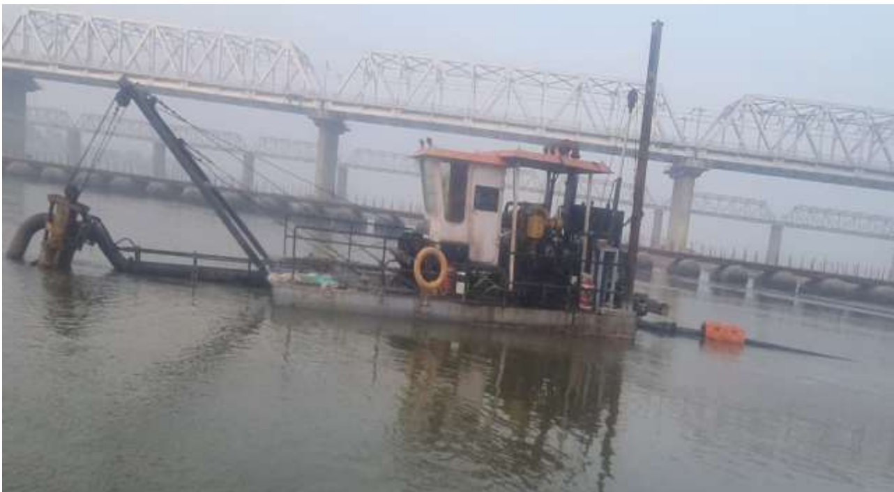
Figure 22: Additional Dredger Machine as per Requirement
