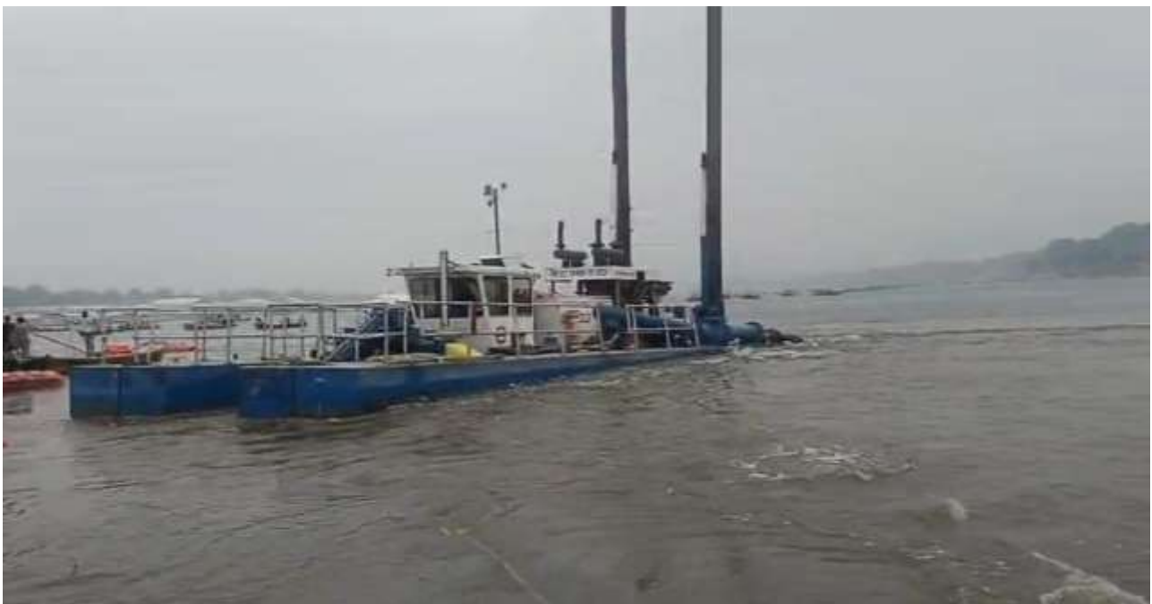
Figure 17: Dredger Ellicot Facing Strong Current in river Ganga during dredging
