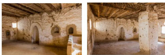
Figure (3) illustrates the mosque is built of mud bricks and is distinguished by its architectural simplicity. It contains a pulpit and a mihrab
