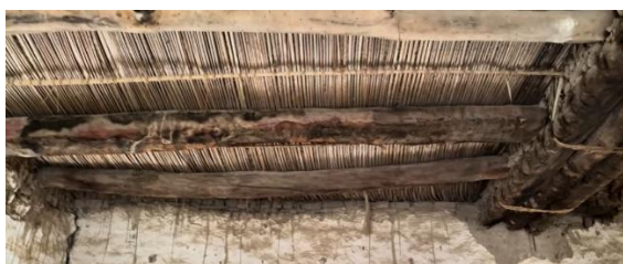
Figure (7) illustrates Palm fronds and spathes (the inner stalks of the fronds) are used for roofing
