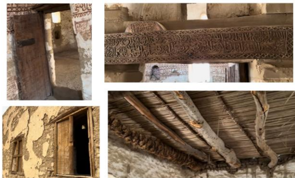
Figure (8) illustrates Tamarisk and palm wood were used in the manufacture of doors, windows, and roof beams
