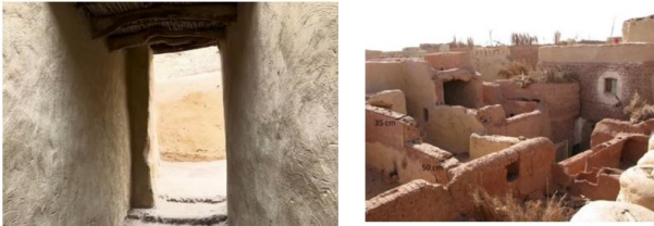
Figure (5) illustrates Buildings are characterized by thick walls that insulate against heat
