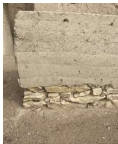
Plate 6: Mud Wall Stone Foundation. Photo by authors.
